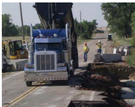
Culvert and roadway repair work in progress
