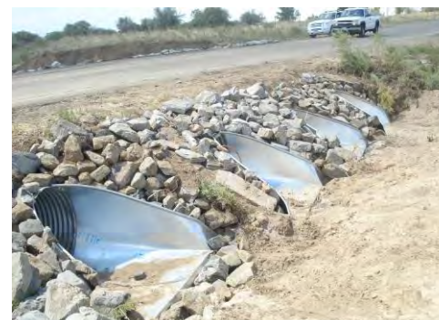
Completed culvert repair to increase conveyance
