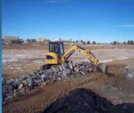
Low-Flow Channel Stabilization
