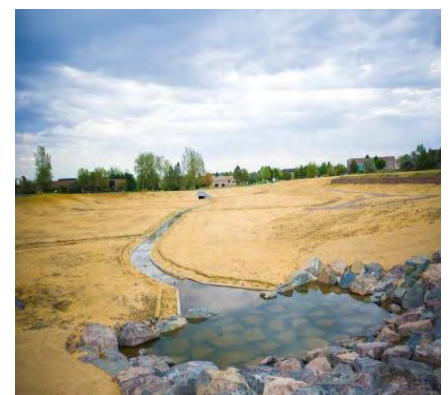
Lone Tree Creek Regional Pond L-2 located north of the Centennial Airport provides regional flood detention and water quality treatment for a developing area
