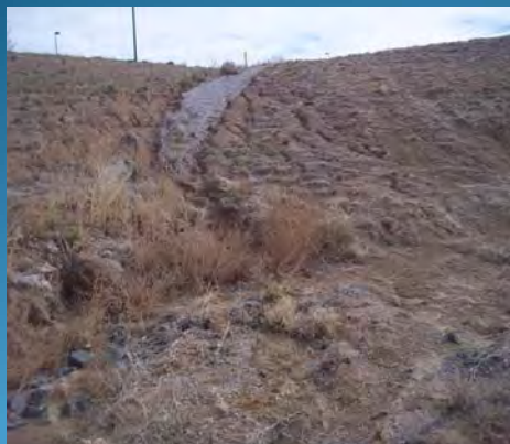
Embankment Erosion Before
