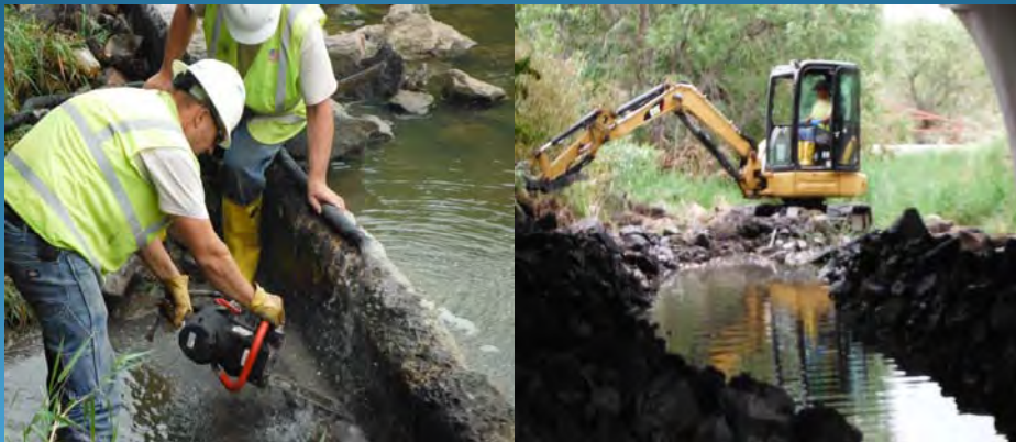
Sectioning Concrete Dam Wall
