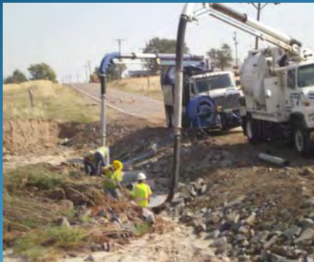
Clean Sediment from Pipe
