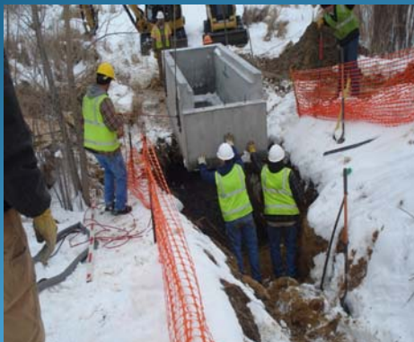
Setting Precast Stilling Basin
