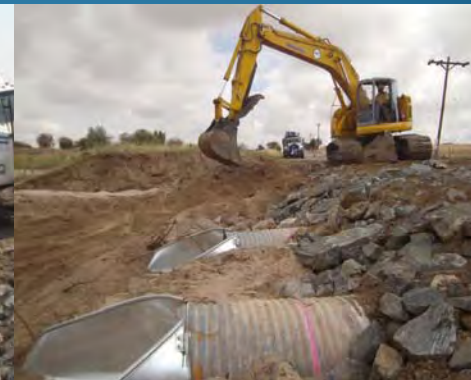
Import Fill Material and Reconstruct Embankment
