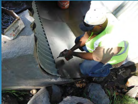
Corrugated Metal Culvert Repair at Jamison and Willow Creek
