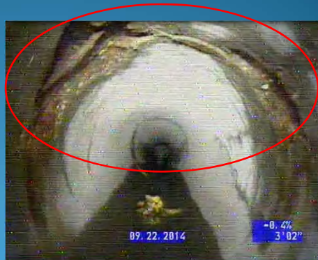
Utility Bore Intrusion at 7902 Vincennes Way
