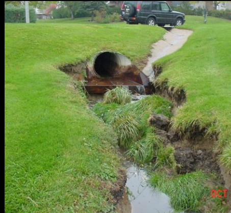
Willow Creek MNA-identified remedial project in the Willow Creek subdivision
