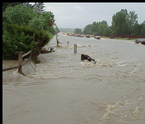
Flooding problems on Arapahoe Road require a CIP project for Little Dry Creek flows
