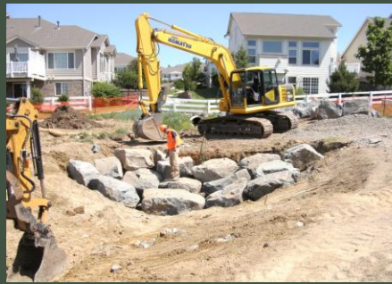
Smoky Hill Detention Pond & Trickle Channel Sediment Removal
