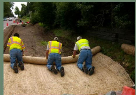
Erosion control blanket installation
