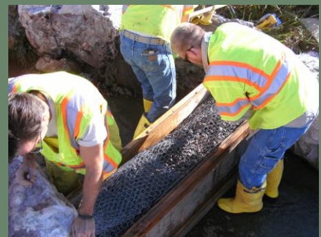
Installing temporary check dams
