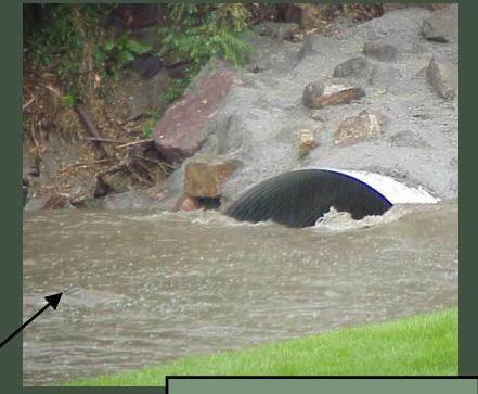
South side of Arapahoe Road
