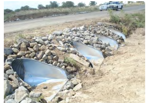
Completed culvert repair to increase conveyance
