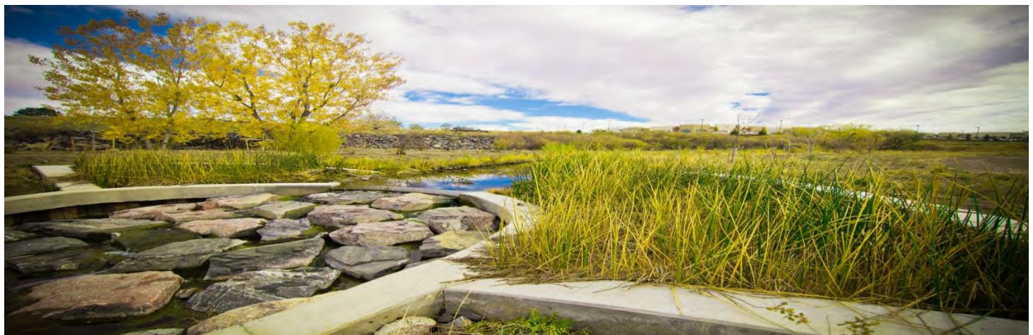
Drop structure in Cottonwood Creek, a component of the regional stream stabilization efforts to minimize transport of sediment to Cherry Creek and the Reservoir
