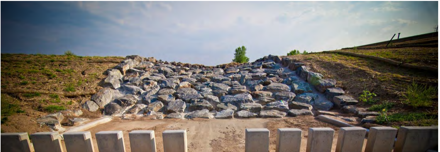
This grouted boulder rundown into Regional Pond D-2 with concrete baffle energy-dissipater blocks provides stability during high flow events in Dove Creek
