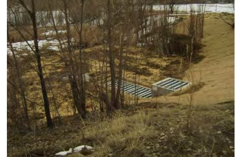
Completed WQ outlet structure at Mexico Pond
