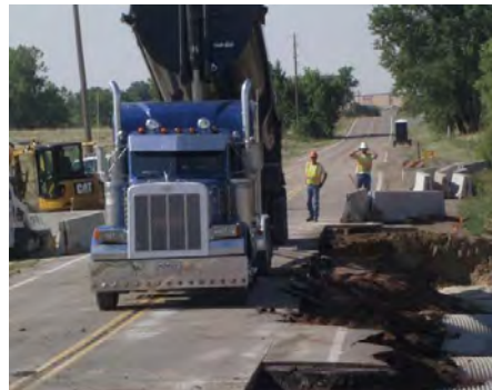
Culvert and roadway repair work in progress
