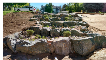
Award-winning runoff design for an outfall to Willow Creek, downstream of Englewood Dam.
