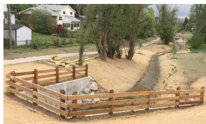
Advancing the tunneling equipment under Yosemite. Completed Xanthia Street culvert for Little Dry Creek flows.
