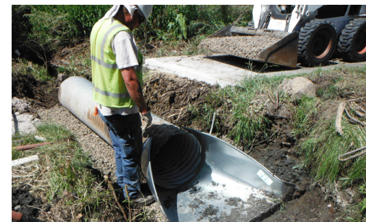
This trail culvert that conveys storm and flood flows to the nearest drainageway was damaged and required replacement, with the addition of a flared end section that provides a preferred path for the runoff to travel.
