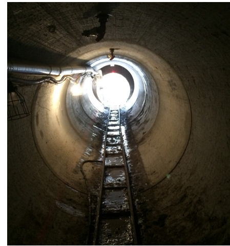
Tunneling equipment used for Little Dry Creek project to install a Yosemite Street culvert.
