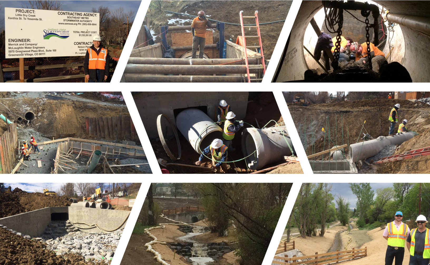
Construction photos of Little Dry Creek channel improvements highlighting the tunneling process used to construct a conveyance culvert under Yosemite Street.
