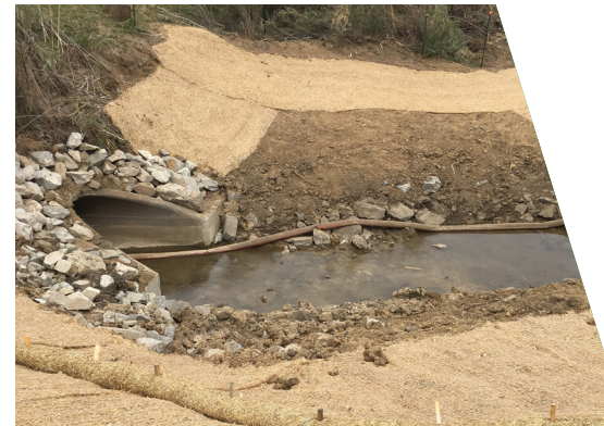
This trail culvert that conveys storm and flood flows to the nearest drainageway was damaged and required replacement, with the addition of a flared end section that provides a preferred path for the runoff to travel.
