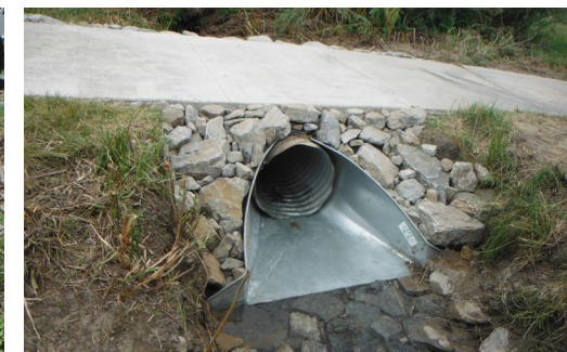
This trail culvert that conveys storm and flood flows to the nearest drainageway was damaged and required replacement, with the addition of a flared end section that provides a preferred path for the runoff to travel.
