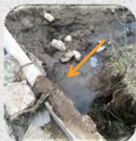
Flows going under drop structure
