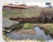
Culvert erosion
