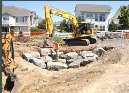
Smoky Hill Detention Pond & Trickle Channel Sediment Removal
