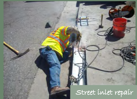
Drop structure grout preparation
