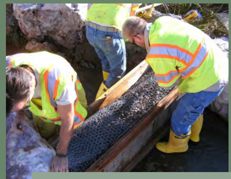
Installing temporary check dams
