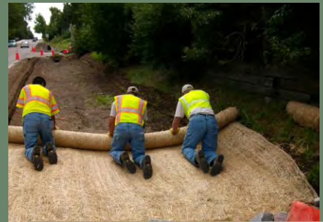
Erosion control blanket installation
