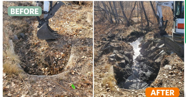
Example Before & After sediment, nuisance vegetation and debris removal to improve flood flow conveyance at outfalls (Above) and storm sewer piping (Below)
