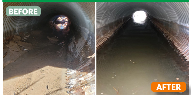
Example Before & After sediment, nuisance vegetation and debris removal to improve flood flow conveyance at outfalls (Above) and storm sewer piping (Below)
